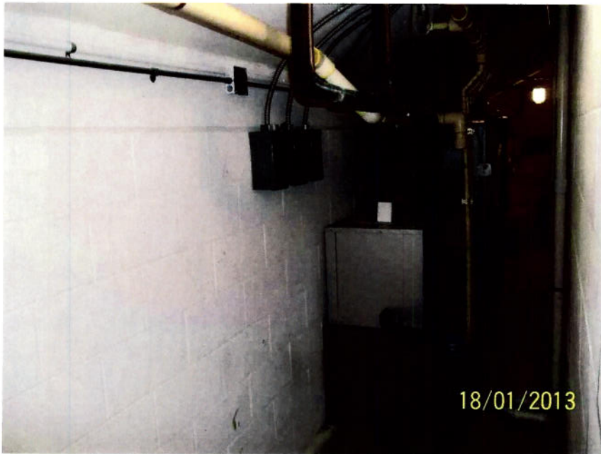
CU-4: Existing unit to be disconnected, sealed off, and left in place to prevent having to disconnect CU-1 for removal of CU-4
