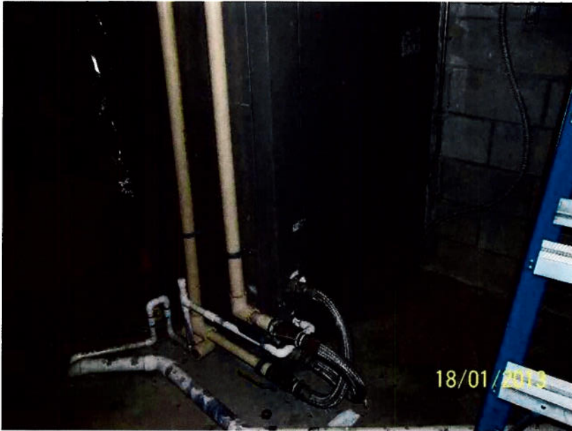
Package Unit#1: Re-circulated coolant water piping connections.
